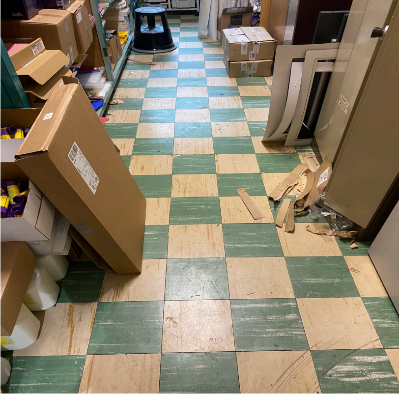
Overall view of the room Aug 2024
